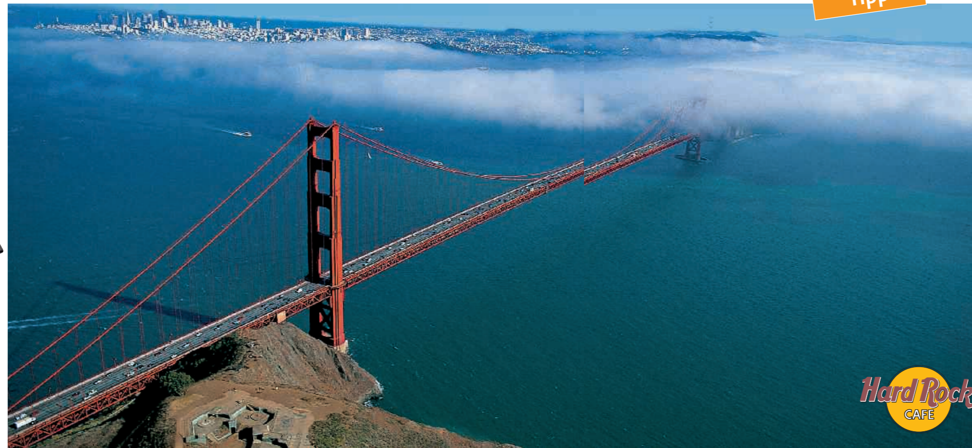
▲ San Francisco, Golden Gate Bridge
